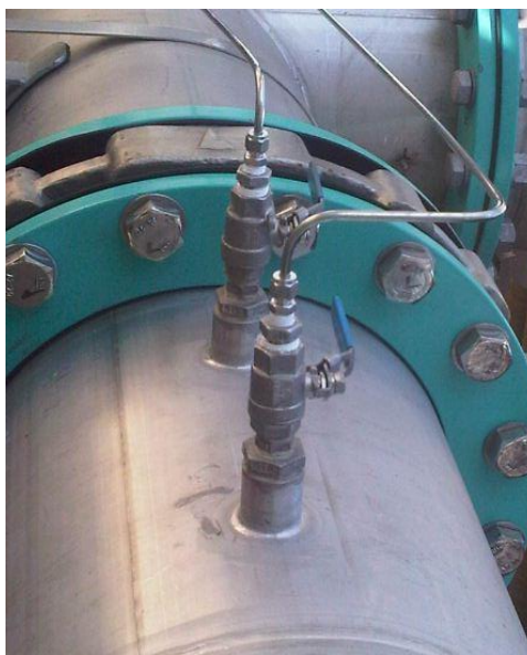
Figure 9 - Ball valve assembly
