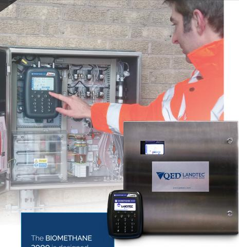
3000 is designed for high accuracy methane and oxygen readings for biomethane applications, providing customers with the peace of mind that at first stage production, they will have quality readings above the 95% methane level and below the 1% oxygen level.
