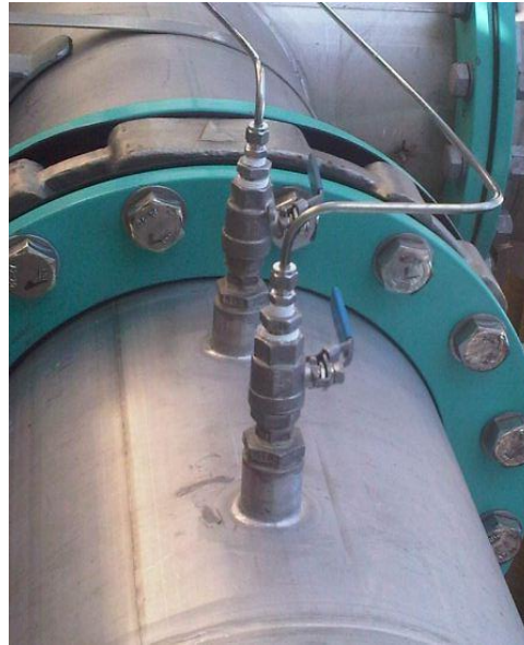
Figure 7 - Ball valve assembly
