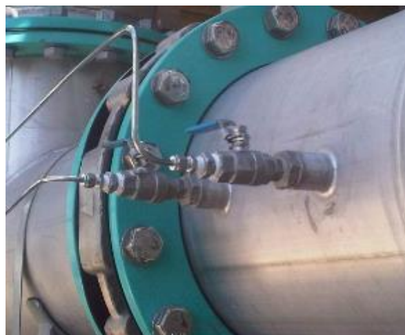
Figure 6 – Ball valve assembly
