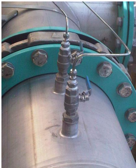
Figure 9 - Ball valve assembly
