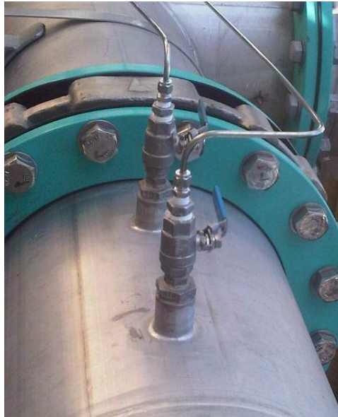
Figure 7 - Ball valve assembly
